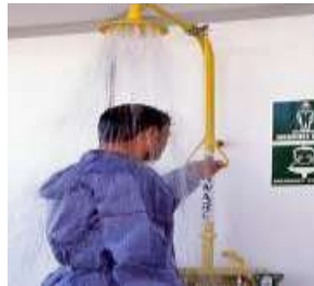
fig 3.3 way of wash during spill
